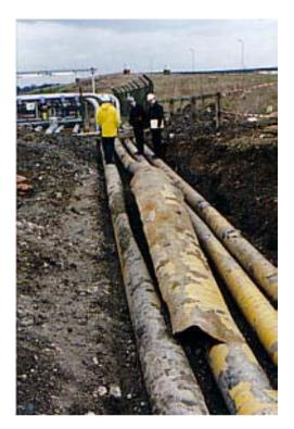
Fig. 1. General View of Surface Pipeline Explosion
